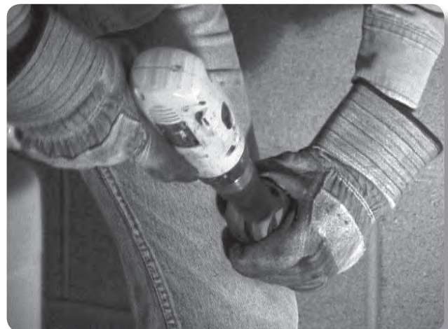
Solution: Using wire brush with power driver
