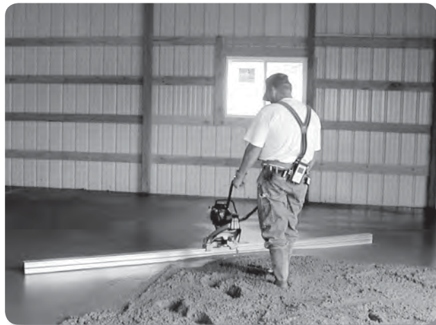
Solution: Motorized screeding
