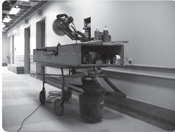
Example: Gurney converted to work table
