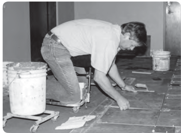
Solution: Laying tile with kneeling creeper
