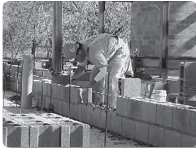
Problem: Laying standard concrete block
