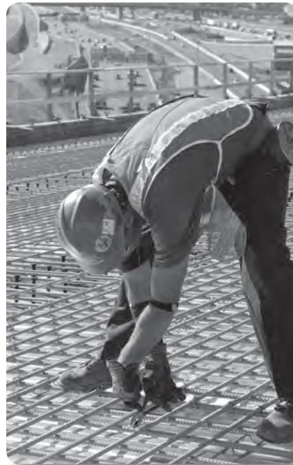
Problem: Tying rebar by hand
