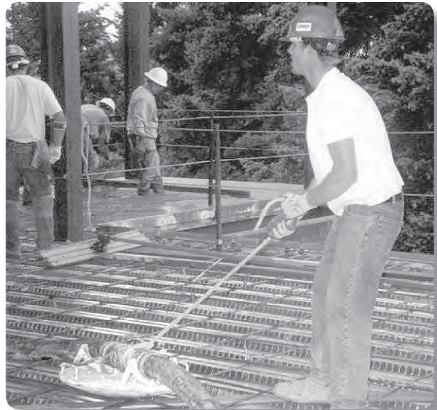
Solution: Pulling hose with skid plate and hook
