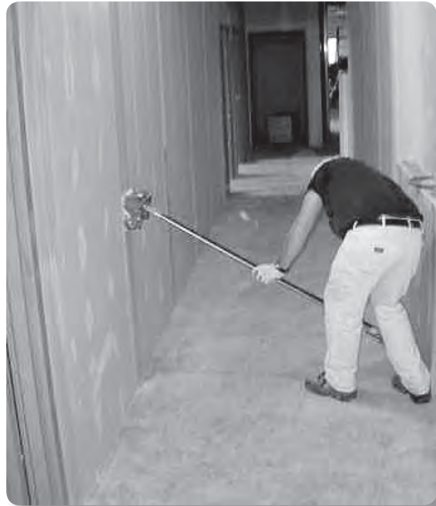
Problem: Hand drywall finishing with mudbox
