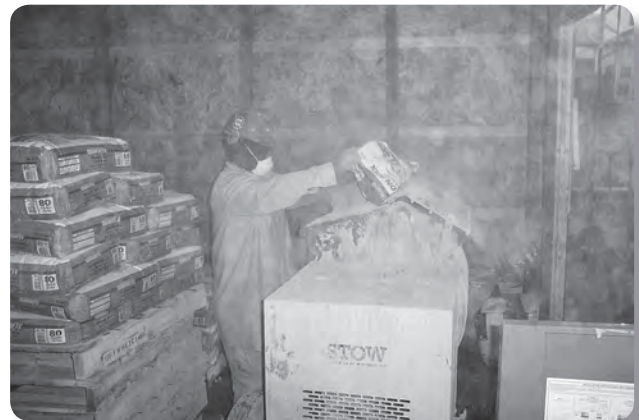
Problem: Traditional method of loading mixer
