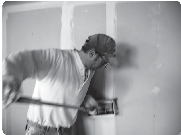
Problem: Hand drywall finishing with mudbox
