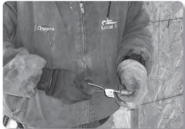
Problem: Brushing copper tube by hand
